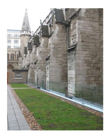
System 17000 AR Sanded Anti-Root is an extremely versatile waterproofing system. It can be used in many situations, including both green roof and Podium deck applications,
